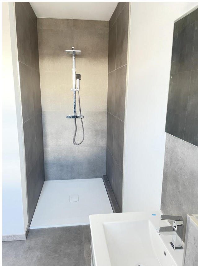
Dusche Gast-WC EG
