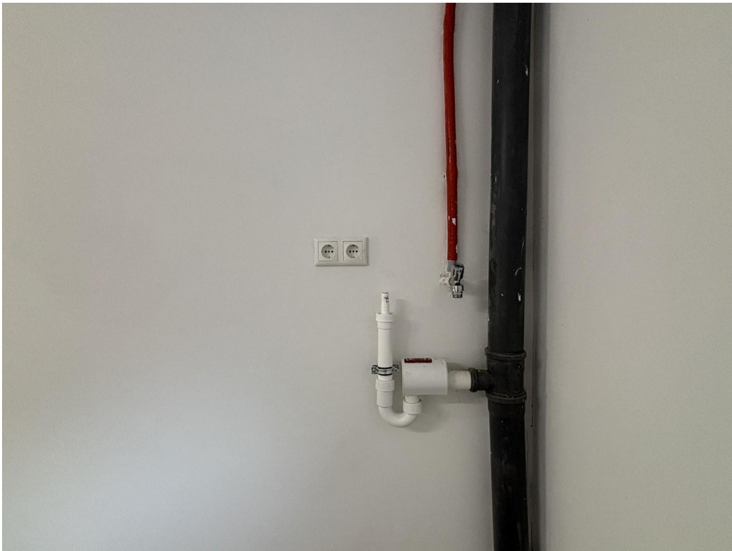
KG Raum 1 (Washing/Storage 1)
