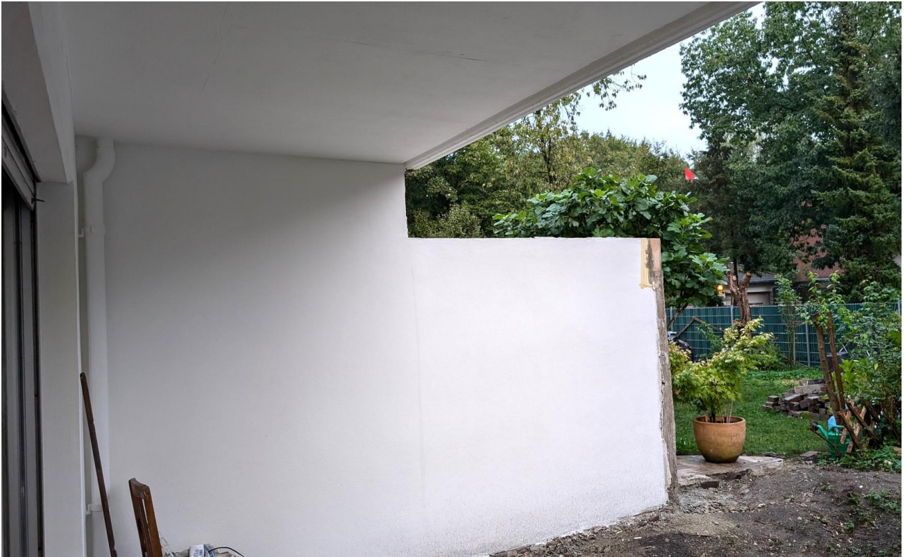
Neue Mauer links
