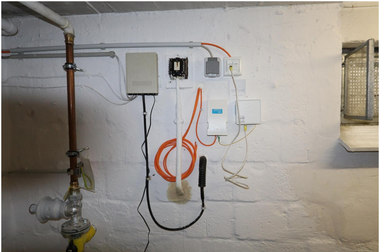
Hausanschlüsse Gas+Glasfaser
