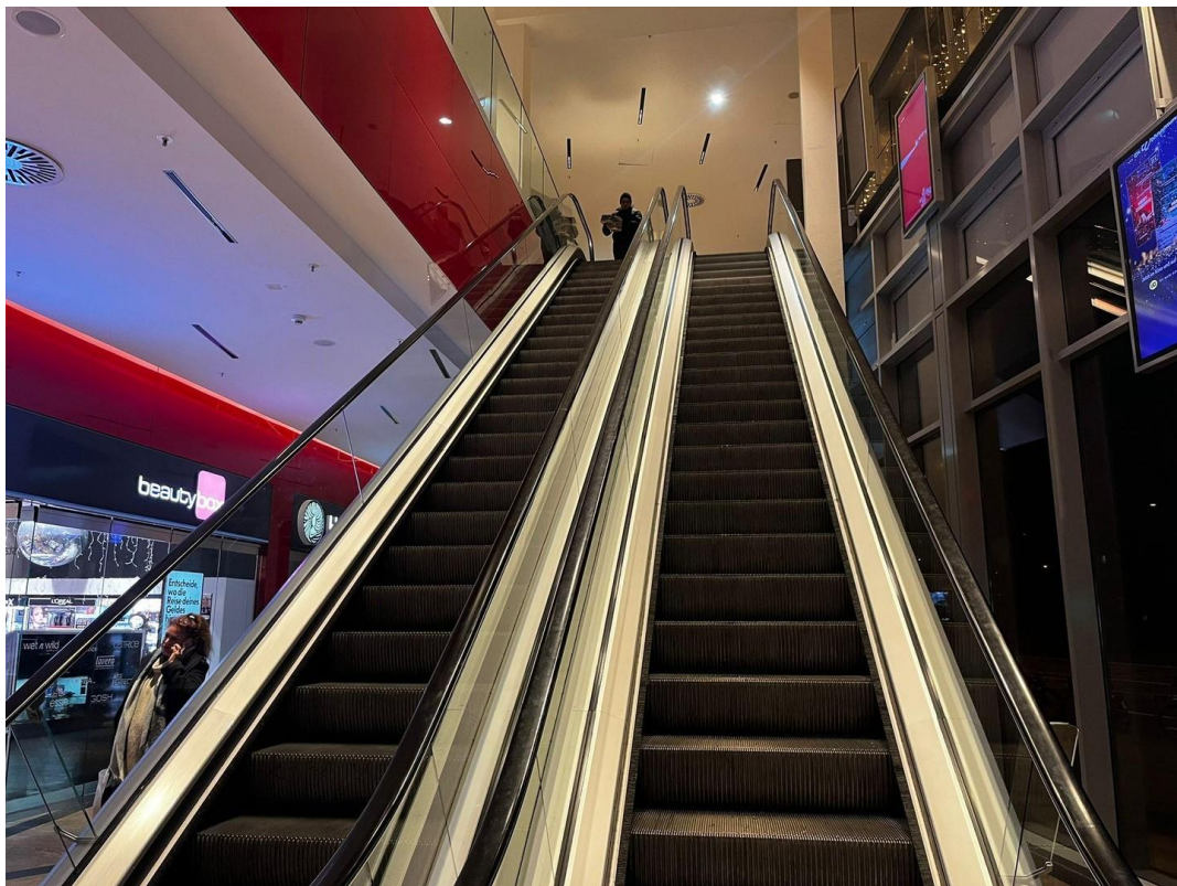
Mundsburg Tower EG
