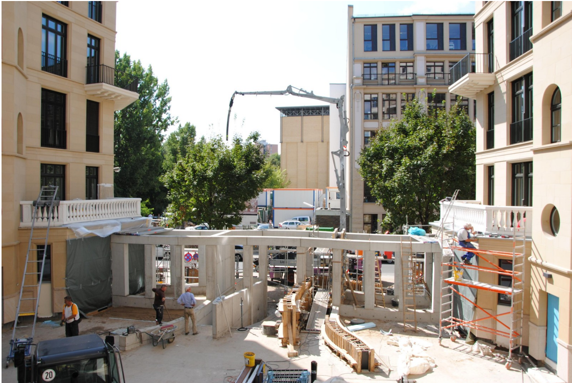
Innenhof Bauphase Fellini 2013
