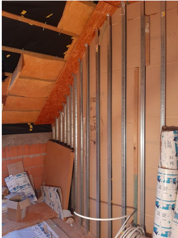
Bad - in Bauphase
