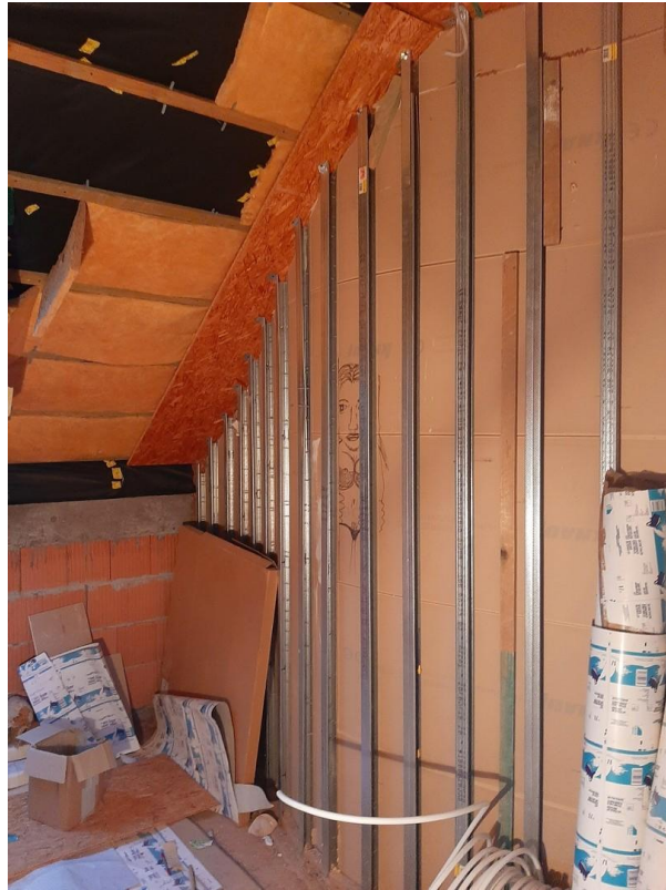
Bad - in Bauphase
