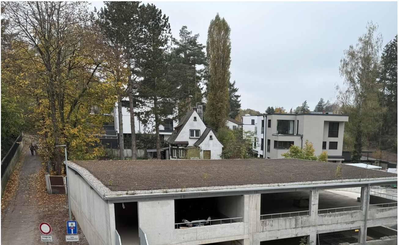
Parkgarage oberes Deck
