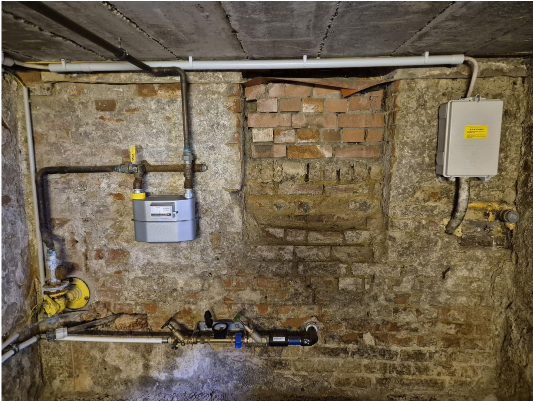
Hausanschlüsse (Gas/Wa./St.)r
