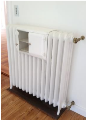
Original cast iron radiator
